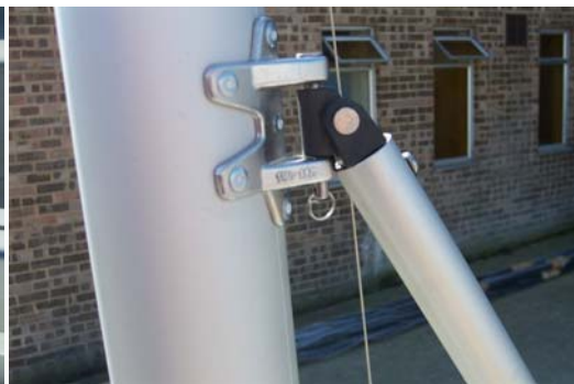
Picture 4.14 Connecting the gnav to the mast
